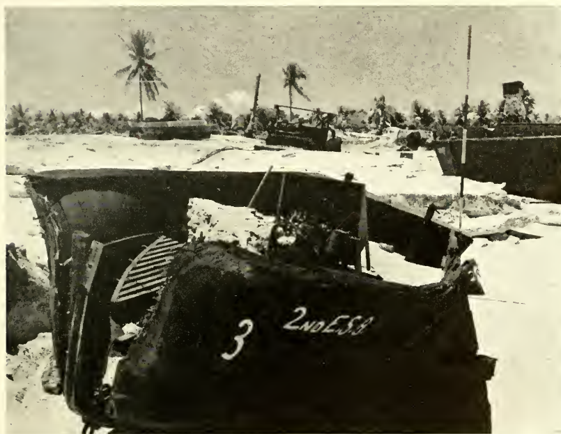
UPPER. Drawing itself up to a height of 15 feet, the first wave produced by the underwater explosion pounds Bikini beach. Note the height-of-water marker pole. LOWER. Backrush from the waves carried 50,000 tons of beach sand into the lagoon. Note erosion visible at right, and the sand-filled boat.
