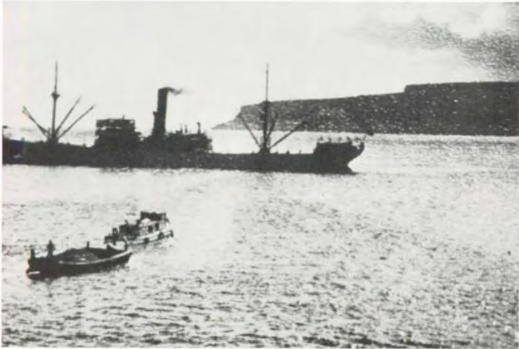
Fig. 11.19. The phosphate ore was transferred to barges by a jump ramp, then towed out to waiting cargo ships. (Photo courtesy of Mark Michael)
