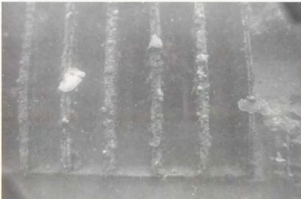
Fig. 9.109. Cargo hold hatch cover beams on the large, unidentified, merchant ship. (NPS photo by Toni Carrell)
