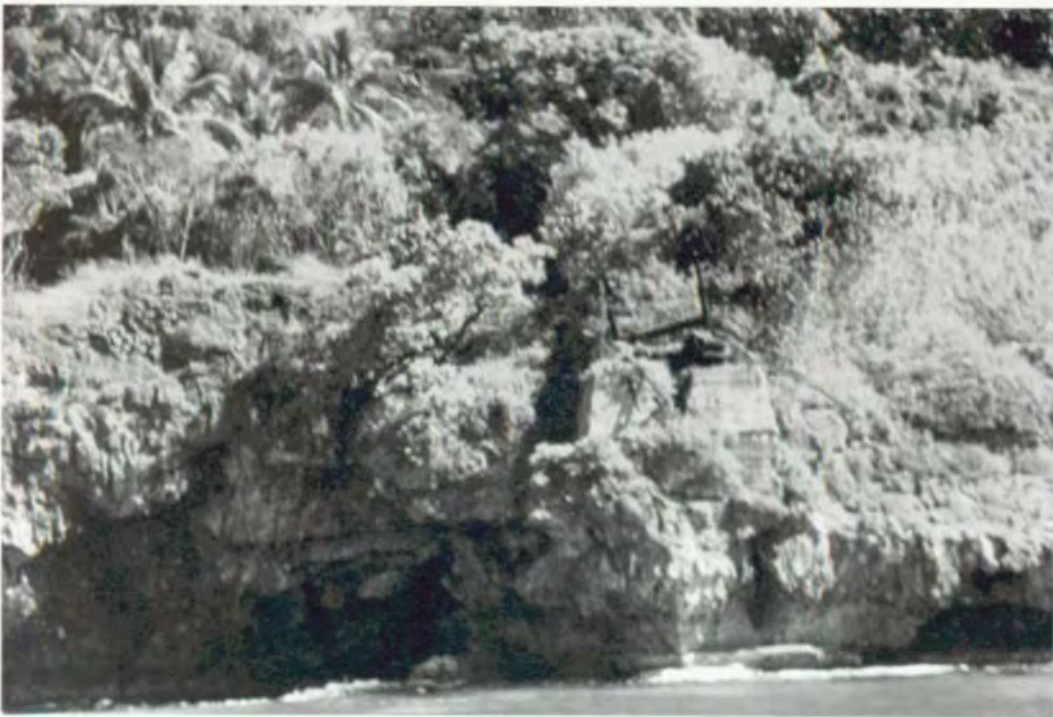
Fig. 11.20. The foundations of a cable tower adjacent to the loading dock are still visible. (Photo by Mark Michael)
