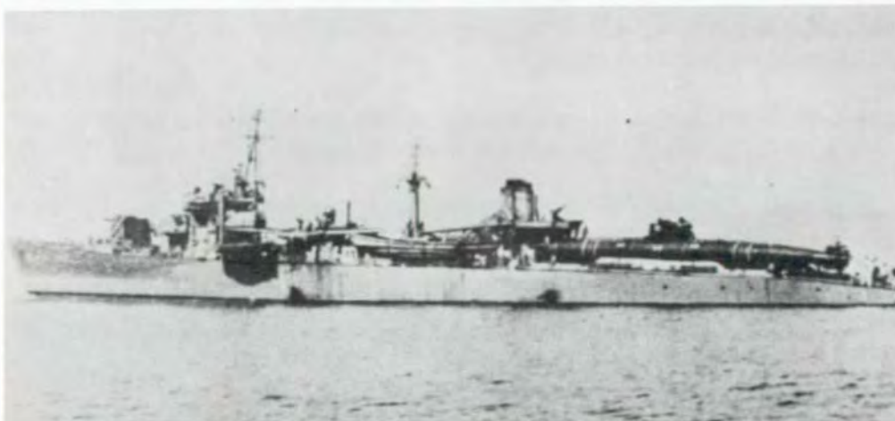
Fig. 9.87. The T.1 fast transports were designed to carry landing craft and amphibious tanks or midget submarines. (Photo courtesy of U.S. Naval Institute Press)
