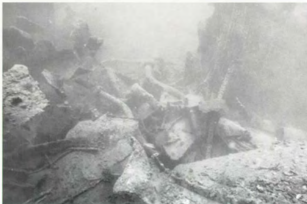
Fig. 9.90. The badly damaged midships machinery space on T.1. (NPS photo by Toni Carrell)
