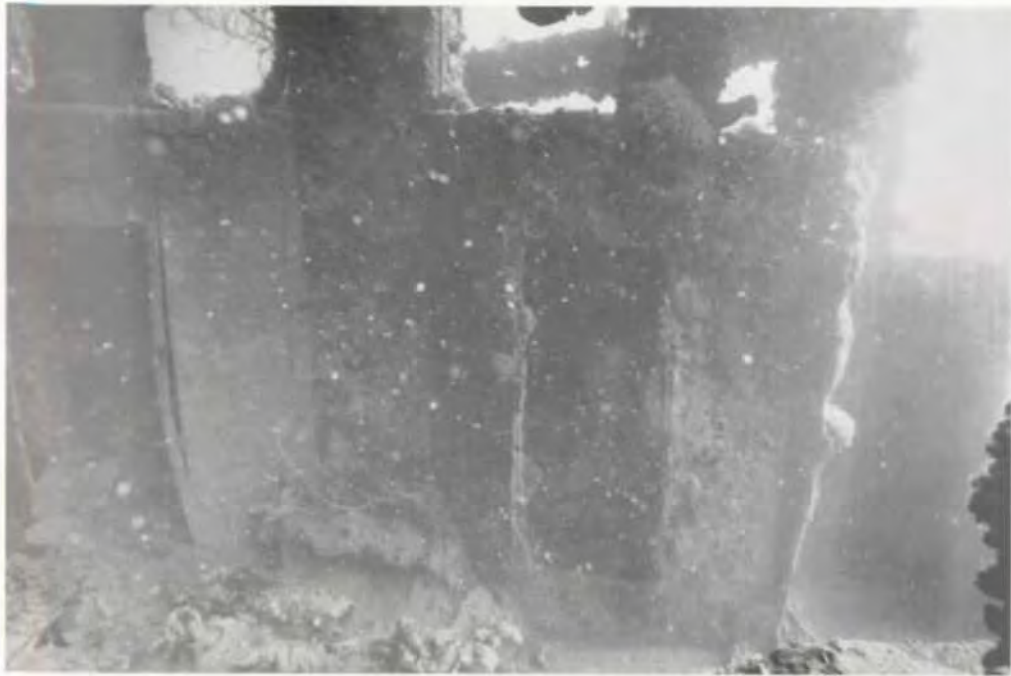
Fig. 9.116. Deck winch house between holds three and four. (NPS photo by Toni Carrell)
