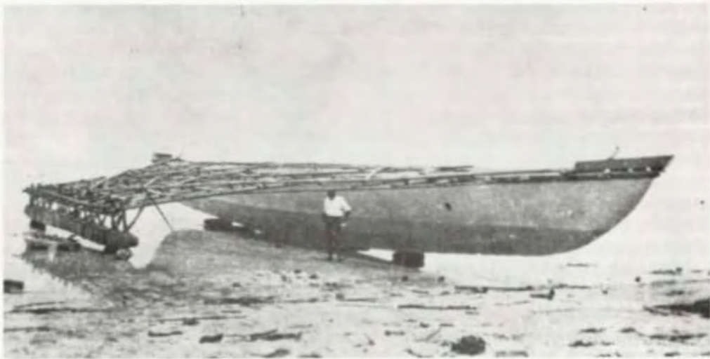
Fig. 5.4. Gilbertese 100-foot baurua under construction at Tabiteuea in 1939. (Photo by H.E. Maude)
