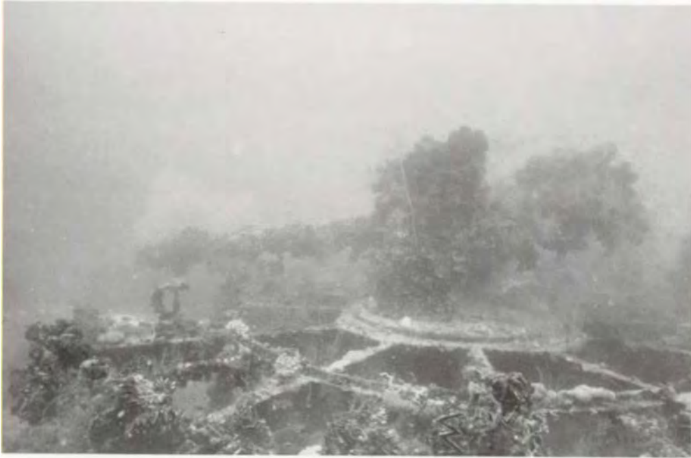
Fig. 9.97. One of two 80-mm, 40-caliber, high-angle guns on IRO. Wooden decking on both the forward gun (seen here) and the aft gun bandstand has deteriorated. (NPS photo by Toni Carrell)
